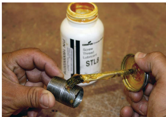
Figure 3-4 Applying conduit lubricant
